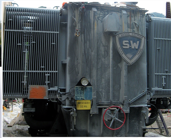
France EDF – Hydraulic power plant Refurbishment TR 40 MVA 225 kV of 1963 realised in 2010
