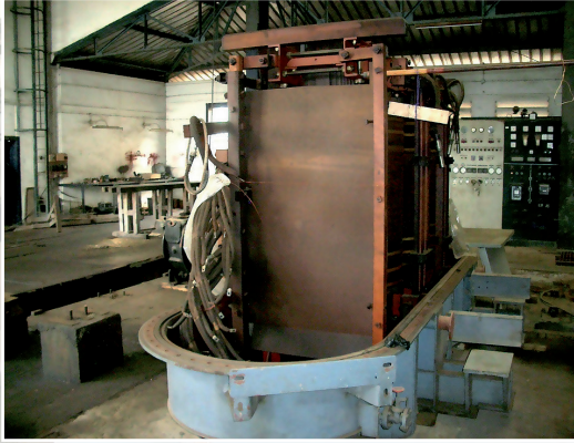
CAMEROON AES SONEL (Refurbishment of TR 10 MVA 90 kV)
